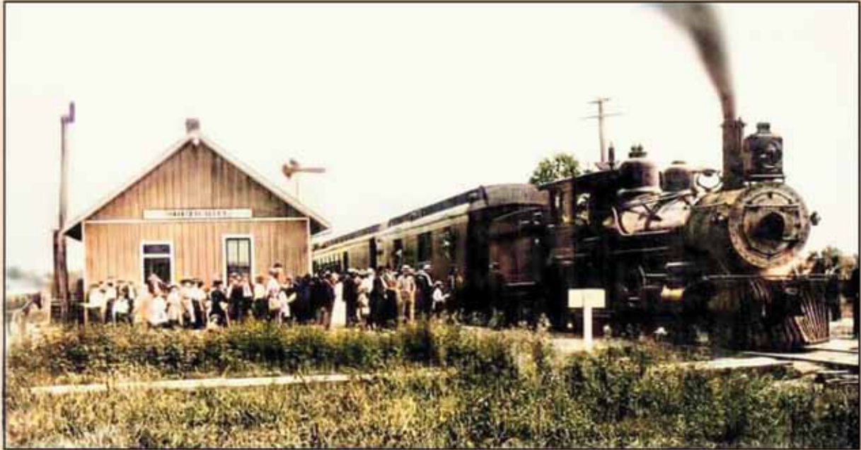
THE OLD TRAIN DEPOT - SOUTH HILL, VIRGINIA
